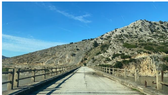
Bridge ober Vjosa River prog. km.3+575 – km.3+750
